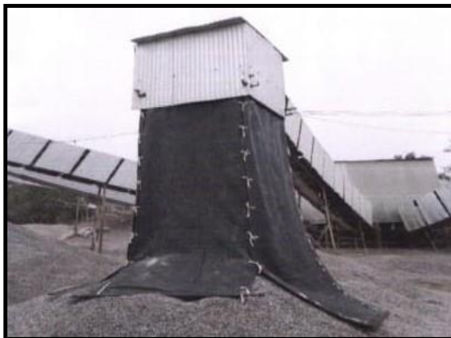
Figure-2: Chute from top of discharge point
